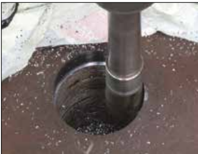
▲ Enlarging a hole
