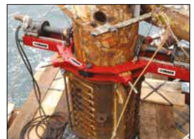
▼ DDU1636 casing pin drilling.
