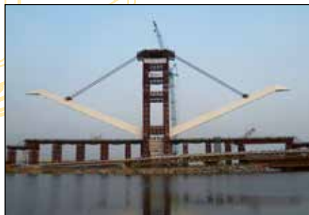
Jacking with high capacity precision control
