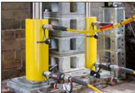
Bridge lifting and launching
