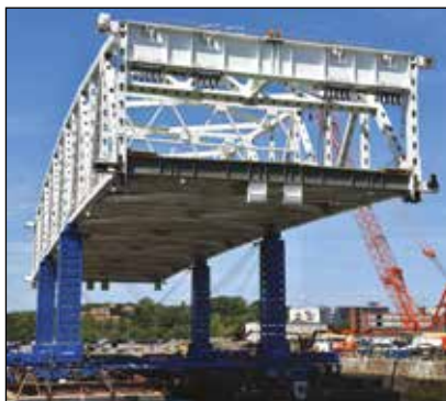
▼ Enerpac Jack-Up System lifts 1500 ton span on Fore River Bridge.
