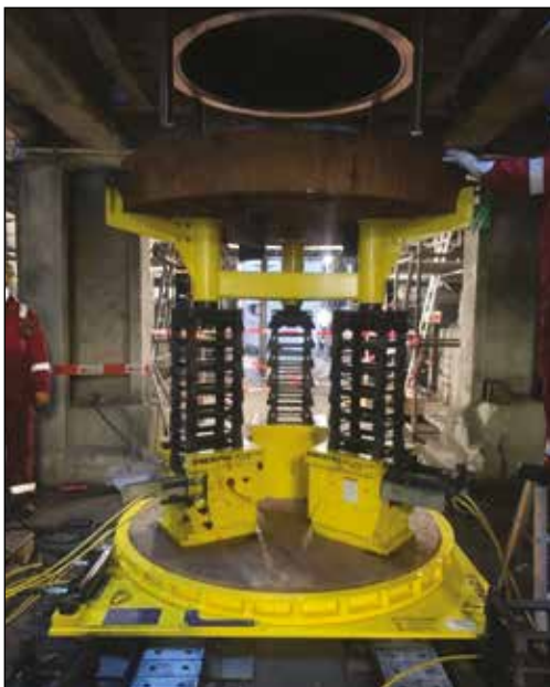
◀ Heat exchanger maintenance job on the piping and condensers at a refinery using a combination of Enerpac Heavy Lifting Technology: SCJ-Series Cube Jacks, the ETT-Series Hydraulic Turntable and LH-Series Low-Height Skidding Systems.
