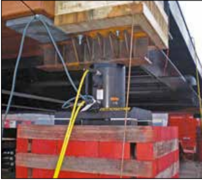
◀ Typical stage-lift application using a custom built Enerpac system to lift the 360 ton Akkerwinde wooden bridge in the Netherlands.
