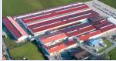
Plant I, Gremsdorf, Germany
