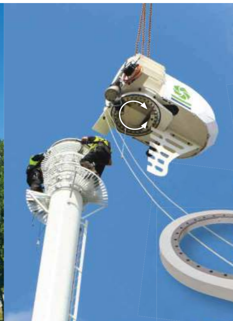
In small wind turbines , slew drives of the SP series are used with or without housings, WD-H or WD-L slew drives are used as yaw bearings or for blade adjustment in plant sizes of 20-150 kW.
