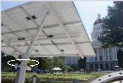
On-roof plant trackers can be rotated with slew drives (here, a slew drive of the WD-L series is used).
